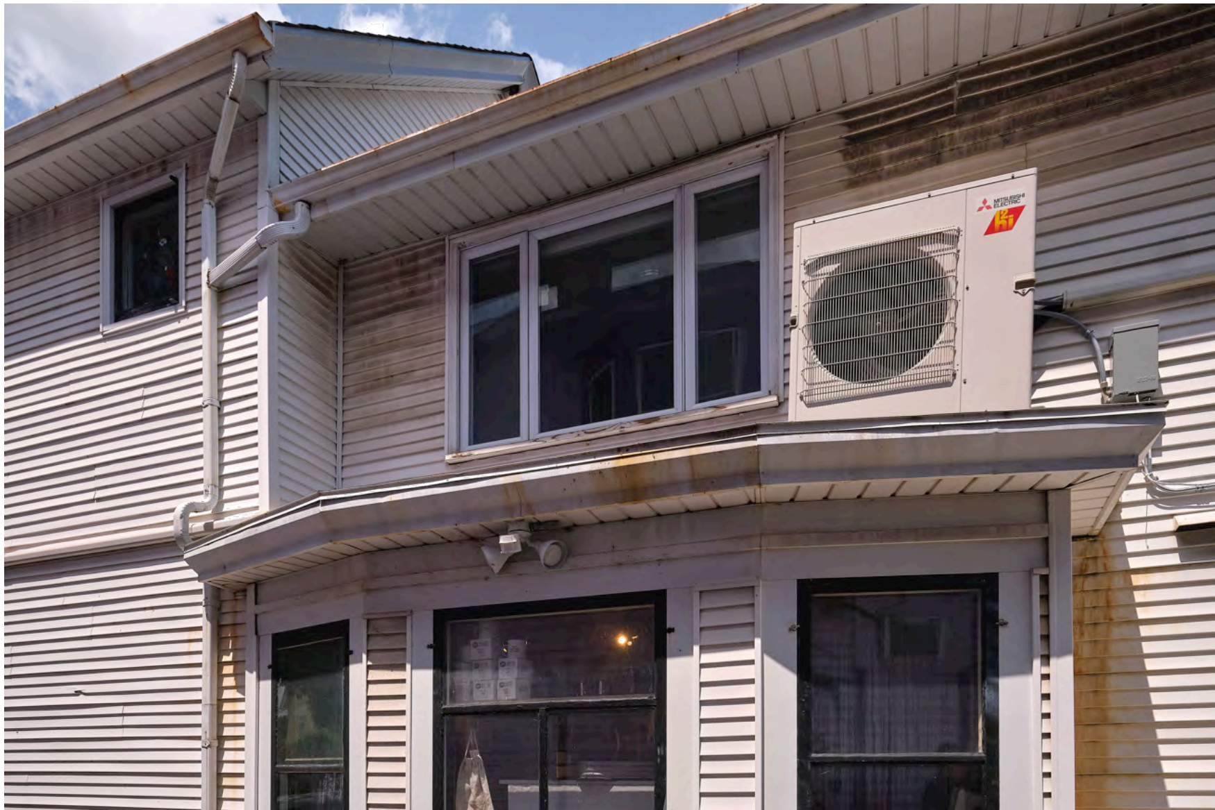
VIEW OF SOUTHERN FACADE SOUTH FROM SIDE YARD
