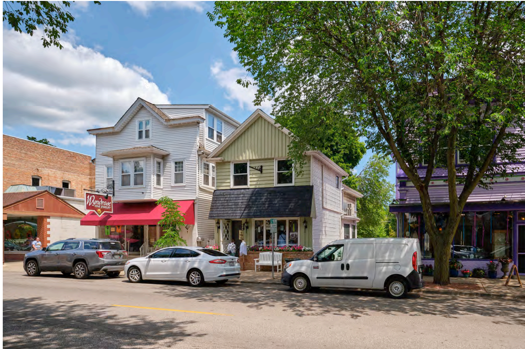
VIEW OF WESTERN FACADE FROM WASHINGTON
