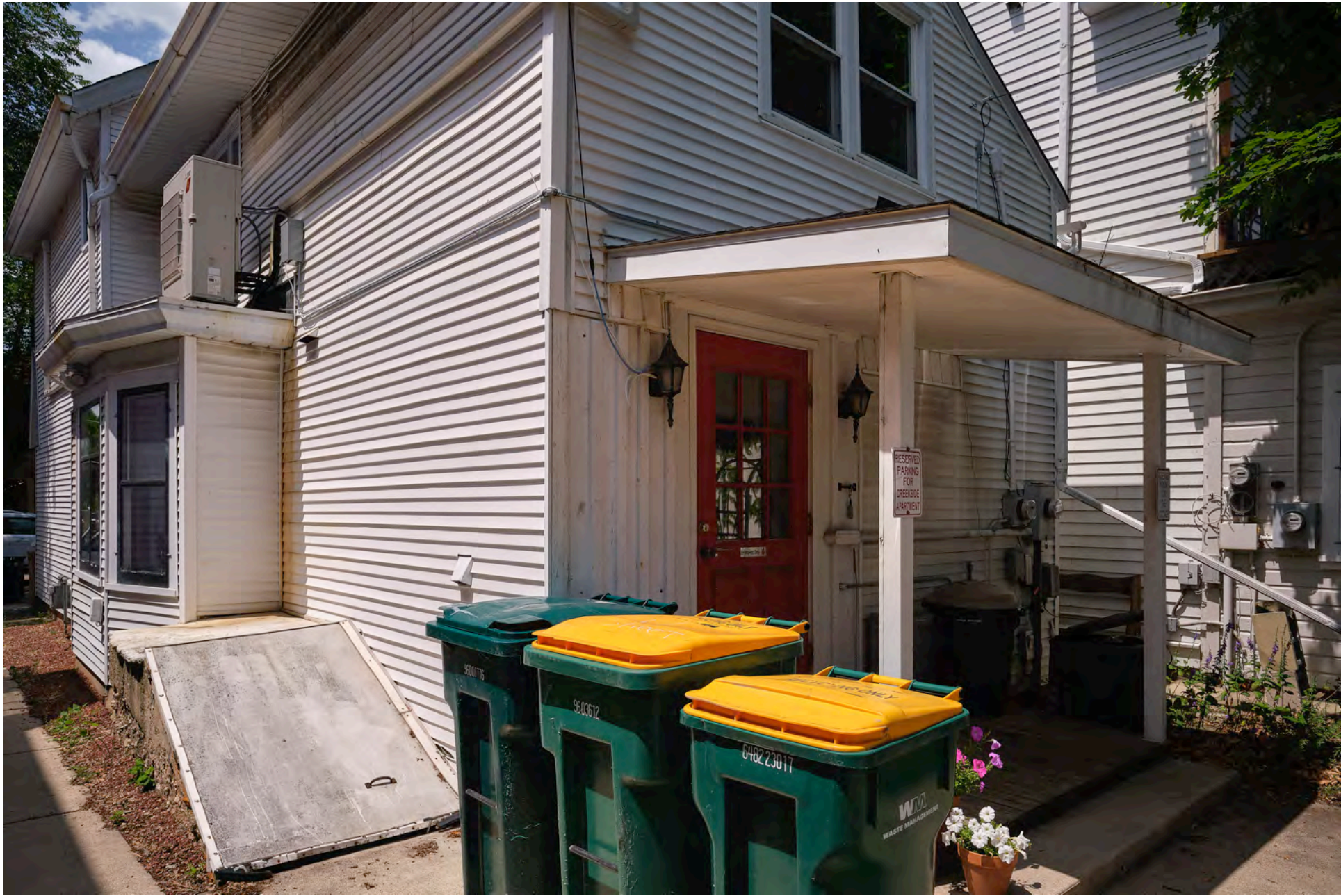
VIEW OF SOUTHERN FACADE FROM SIDE YARD
