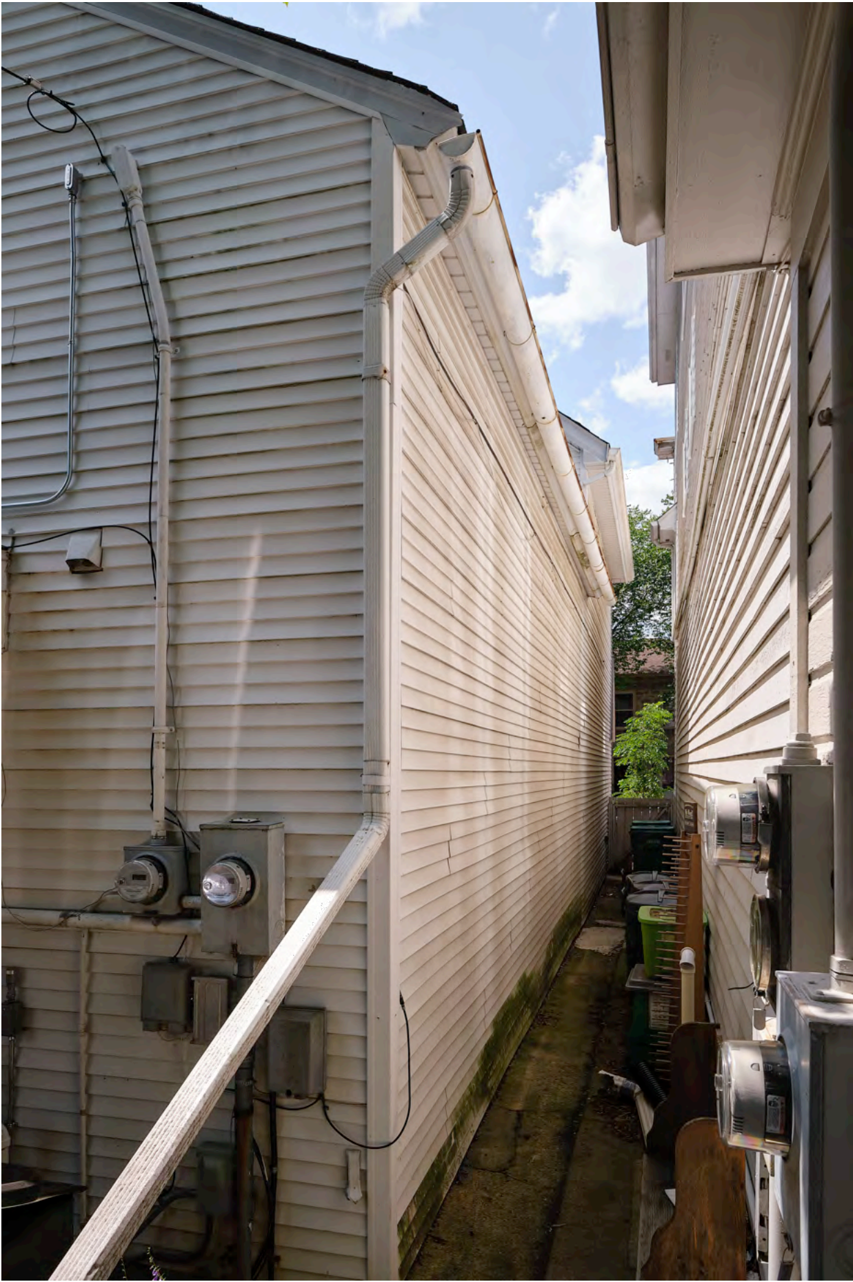
VIEW OF NORTHERN FACADE FROM SIDE YARD
