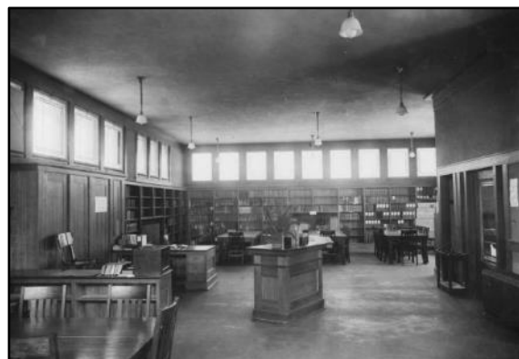
Reedsburg Public Library interior, c.1911
