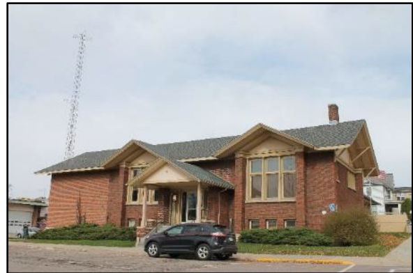
Reedsburg Public Library, 1911 345 Vine Street
