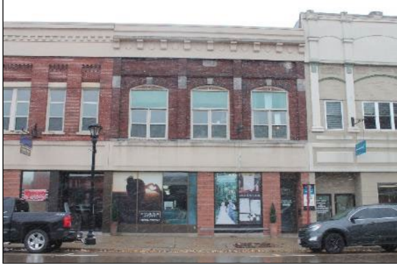
Building, 1902 170 E. Main Street
