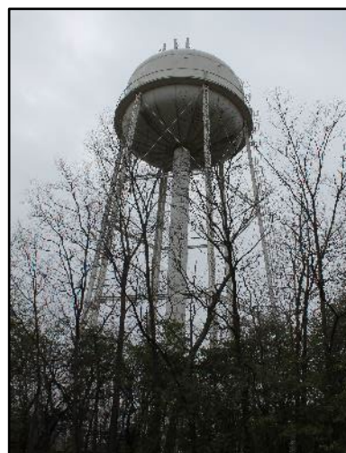
Reedsburg Water Tower, 1973 155 4th Street
