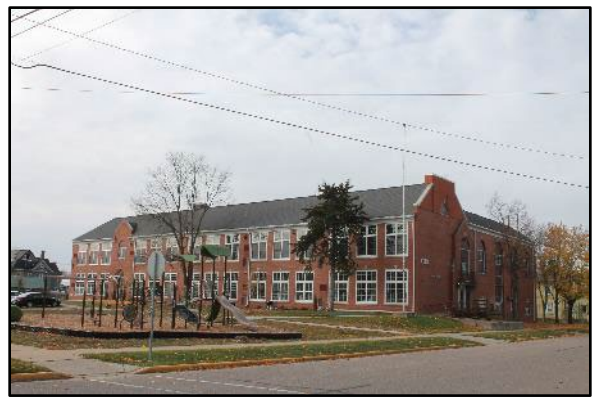
South School, 1937 420 Plum Street
