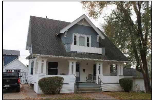
House, 1916 190 3rd Street
