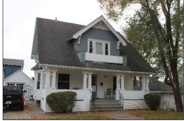
House, 1916 190 3rd Street
