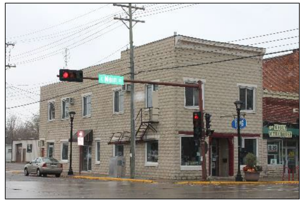
Herman Farber Blacksmith Shop, 1916 46 E. Main Street
