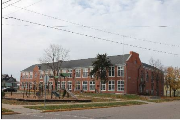
South School, 1937 420 Plum Street
