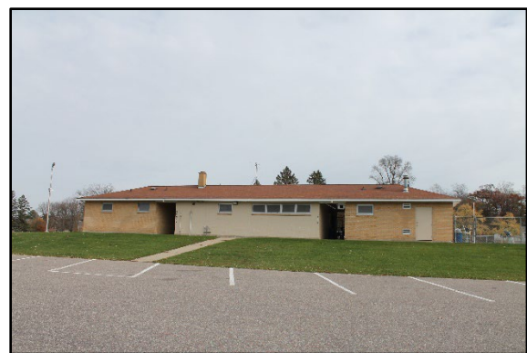
Reedsburg Swimming Pool Bathhouse, 1956 555 N. Webb Avenue
