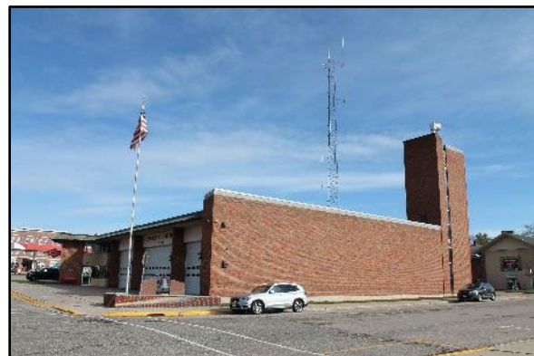
Reedsburg Fire Department, 1971 131 S. Park Street
