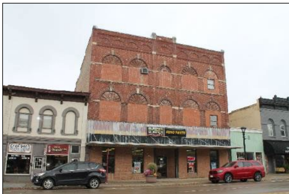
Louis Schulze Building, 1910 139 E. Main Street
