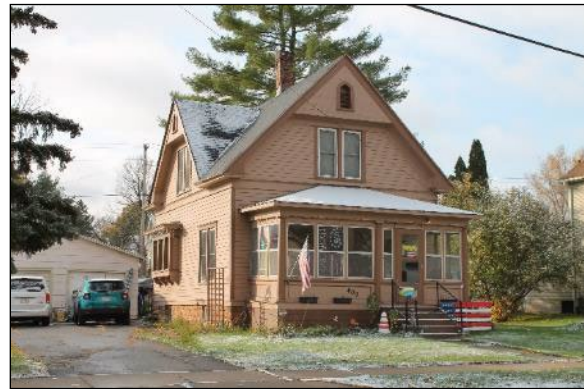
House, 1910 409 W. Main Street
