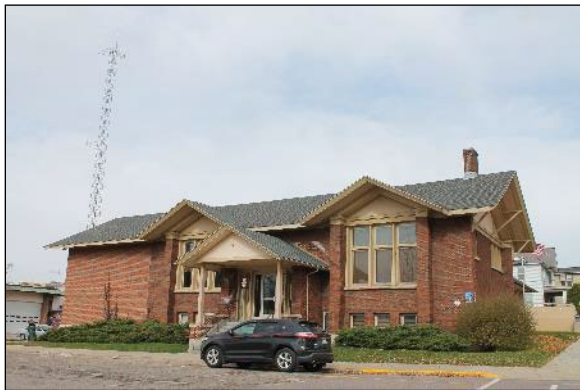
Reedsburg Public Library, 1911 345 Vine Street
