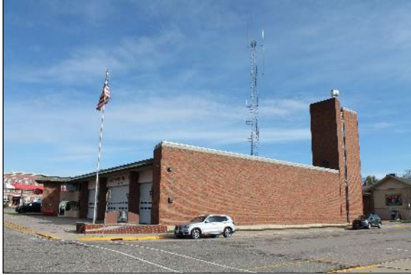
Reedsburg Fire Department, 1971 131 S. Park Street
