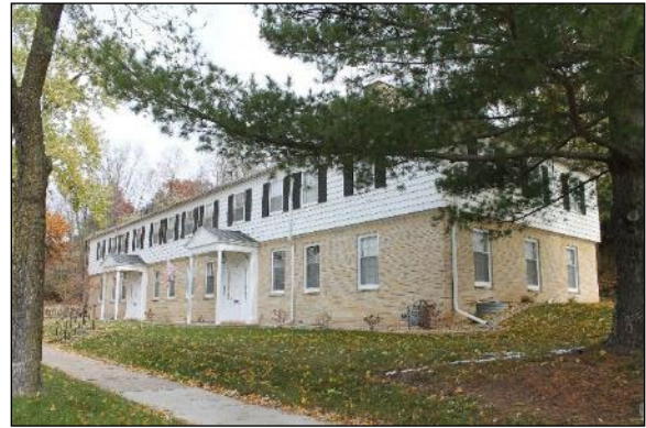
Ramsay Apartments, 1954 400 N. Webb Avenue
