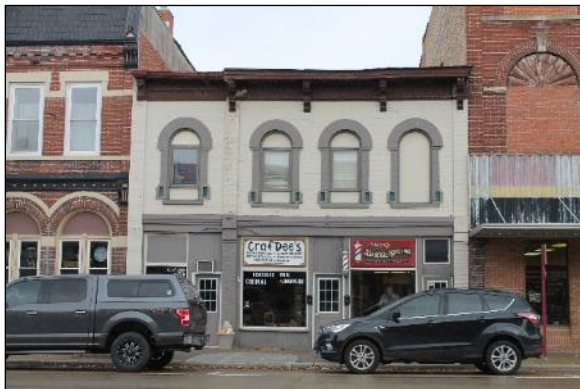
Building, 1873 127 E. Main Street
