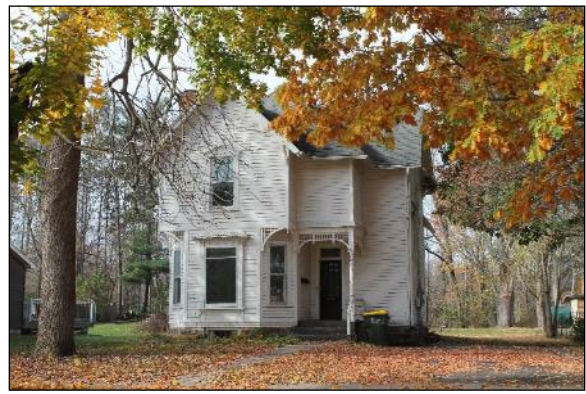
House, 1888 510 S. Park Street
