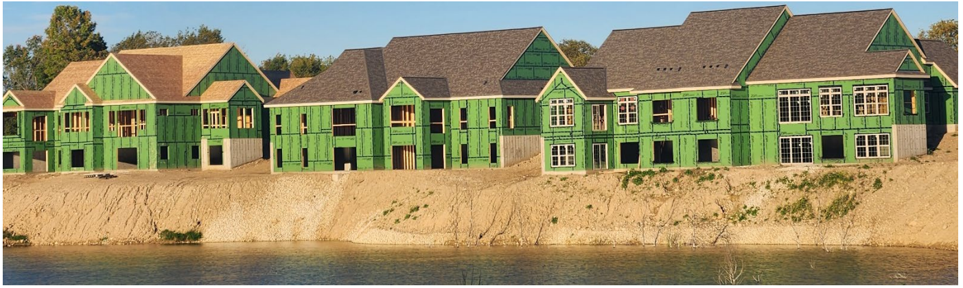
The need for numerous portable ladders cannot be overstated.
