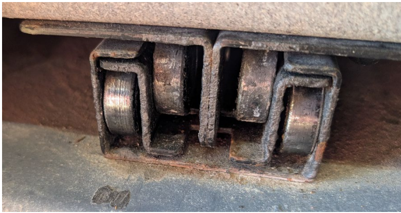
Corrosion was noted on the slide tray hardware.
