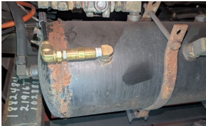
Bolt-on Components Rusting.
