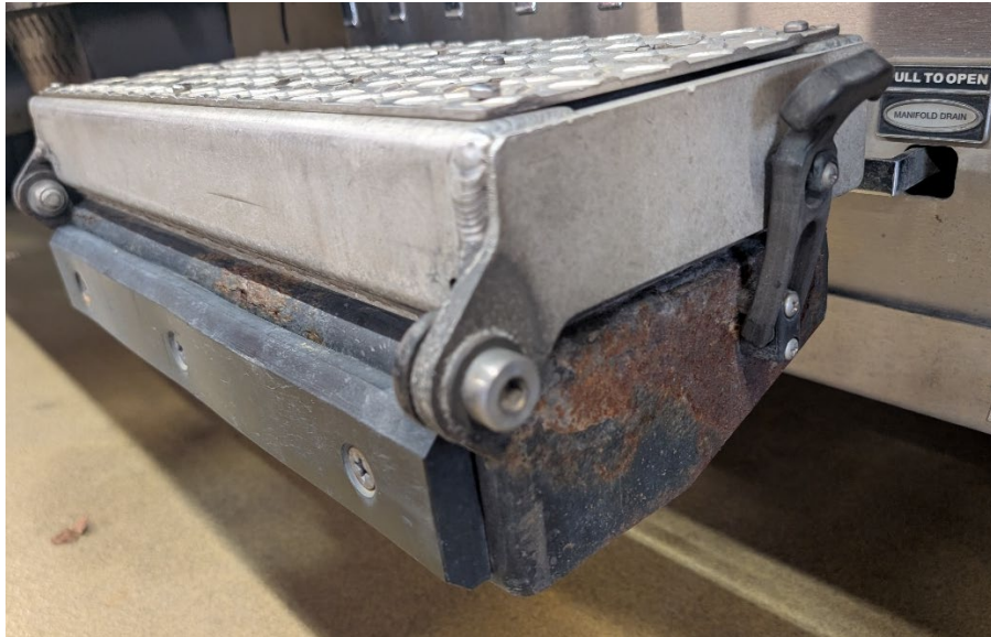
Rust needs to be mitigated on this pump panel step.
