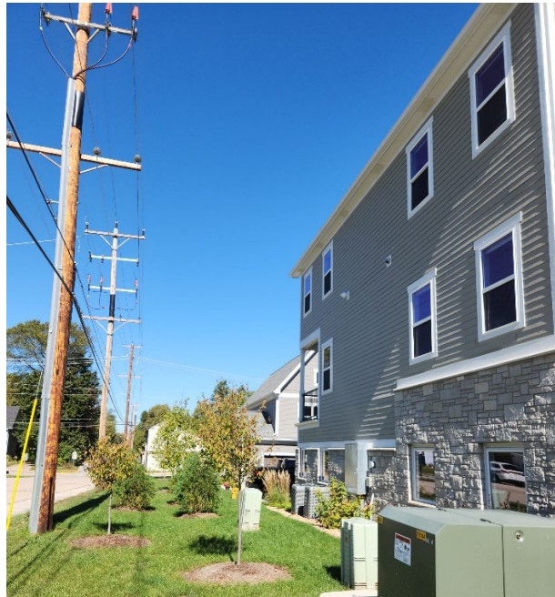
The lack of access for aerial fire apparatus places a greater reliance on portable ladders.
