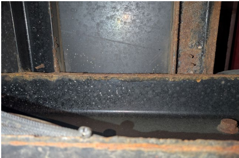
Rust forming on the apparatus sub frame and frame rails
