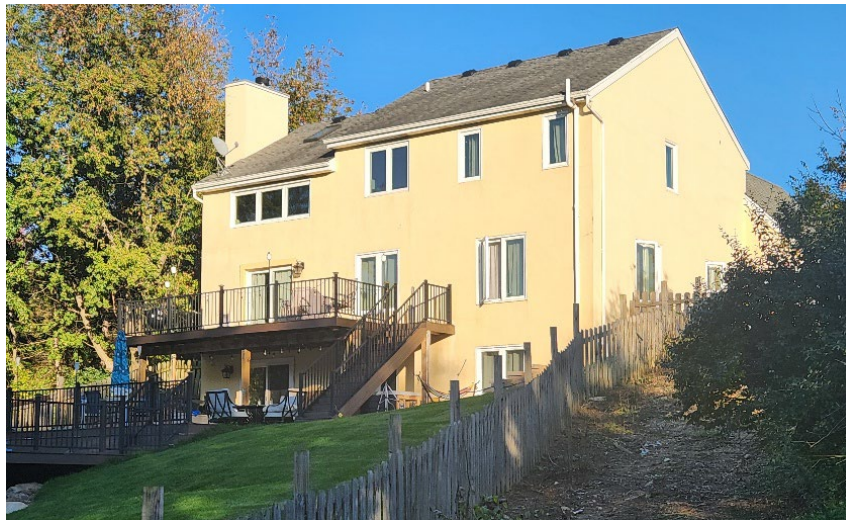
Firefighters trapped on the upper stories would have little chance of survival without multiple 35-foot portable ladders.
