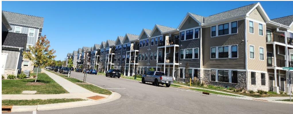
The buildings pictured represent a serious fire problem and a high life safety risk.
