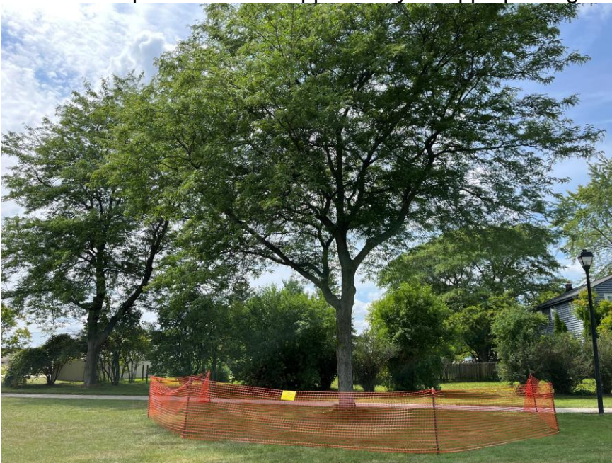
Type 1 Tree Protection Fence at the Canopy Dripline
