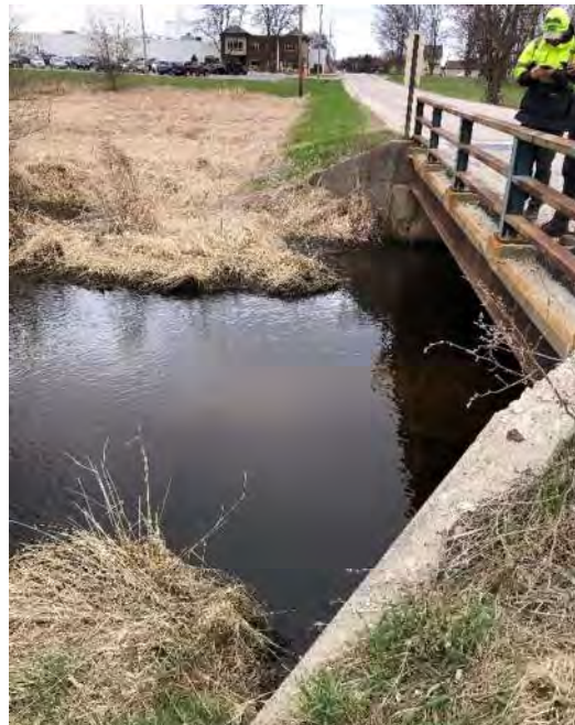
Downstream side of bridge
