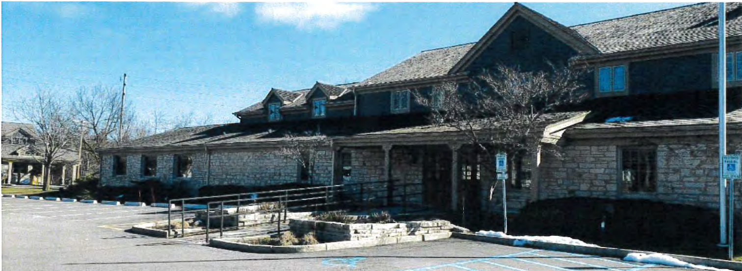
EXISTING WEST BUILDING ENTRY AT NORTH FACADE FACING COLUMBIA ROAD
