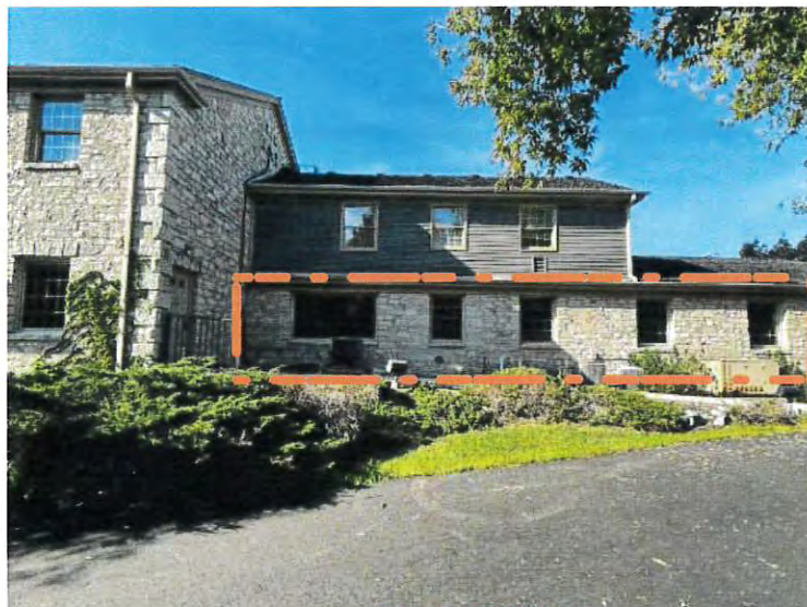
EXISTING SOUTH ELEVATION - STONE TO REMAIN
