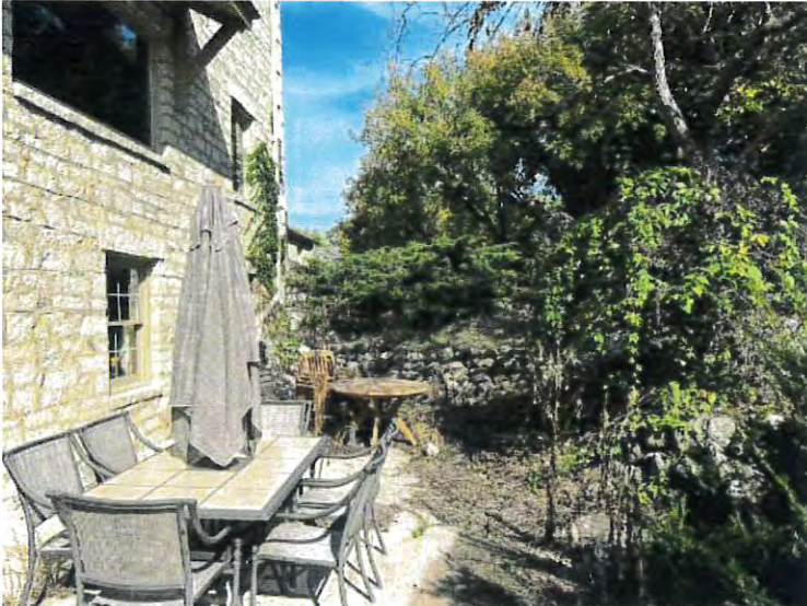
EXISTING LOWER LEVEL PATIO
