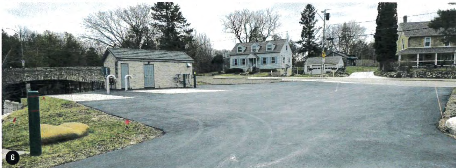
VIEW TO CITY PARCEL FROM SOUTH SERVICE DRIVE
