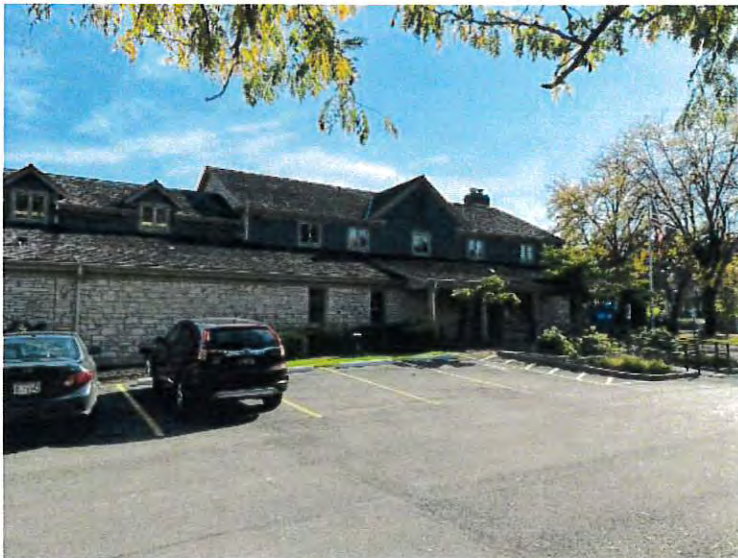
EXISTING NORTH FACADE
