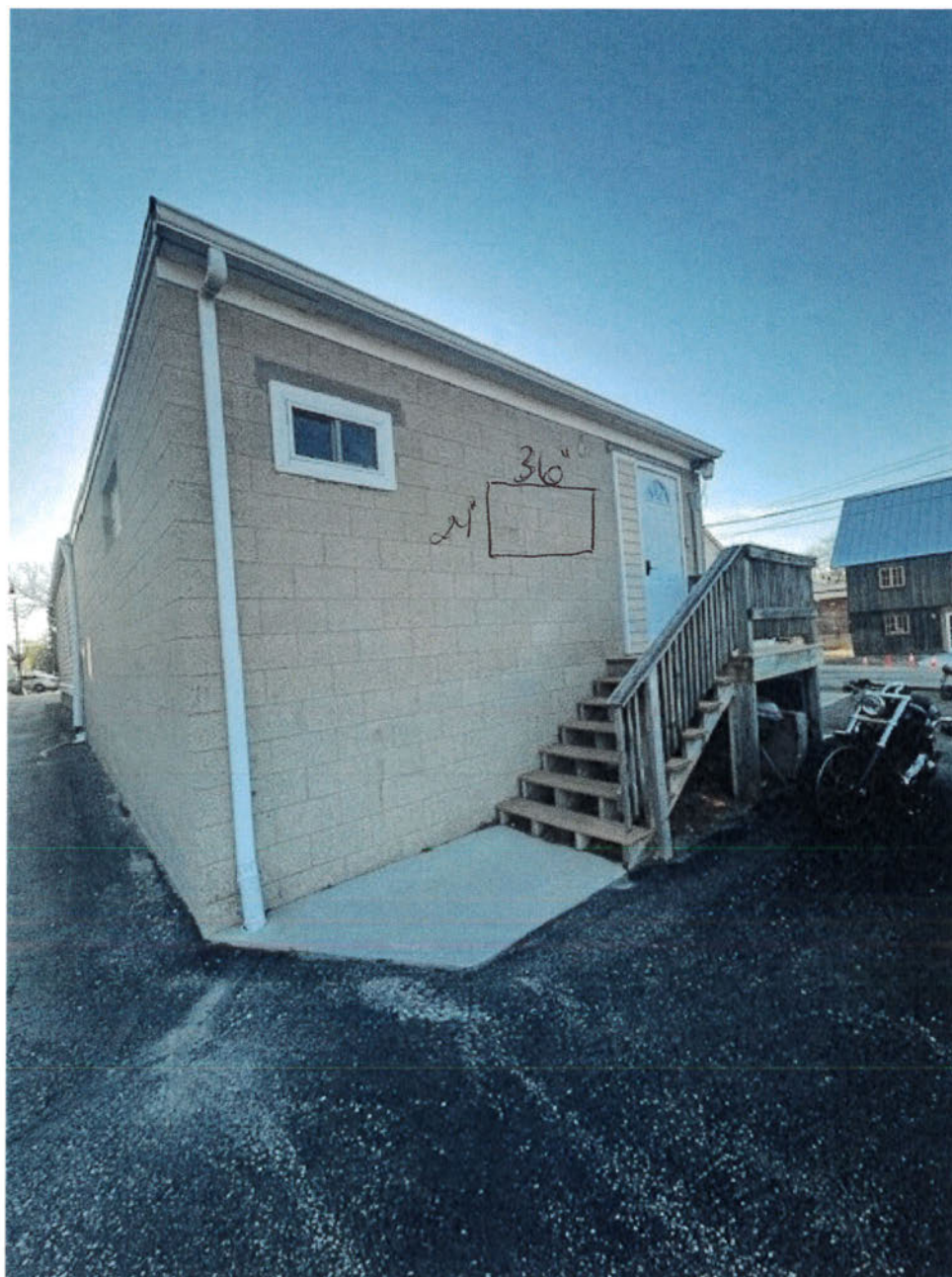
East Side of building
