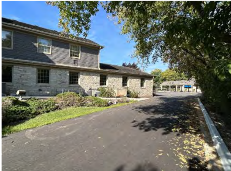
EXISTING SOUTH DRIVEWAY (CEDAR CREEK TO THE RIGHT)
