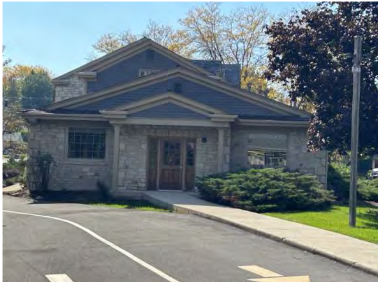
EXISTING EAST ENTRY
