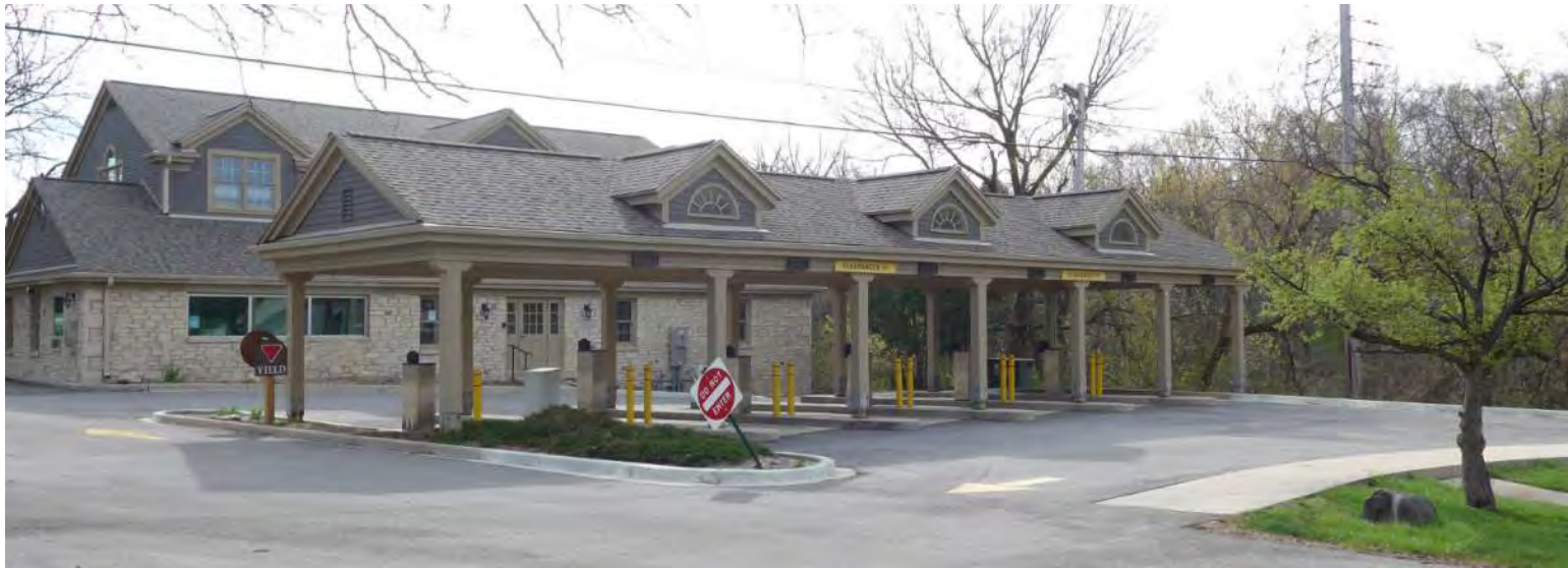
EXISTING DRIVE THRU CANOPY (TO BE REMOVED)
