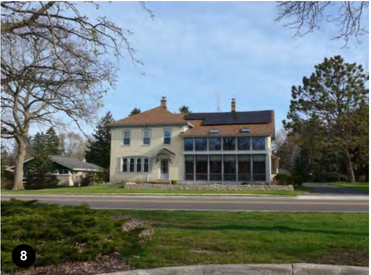
VIEW NORTH AT EAST BUILDING
