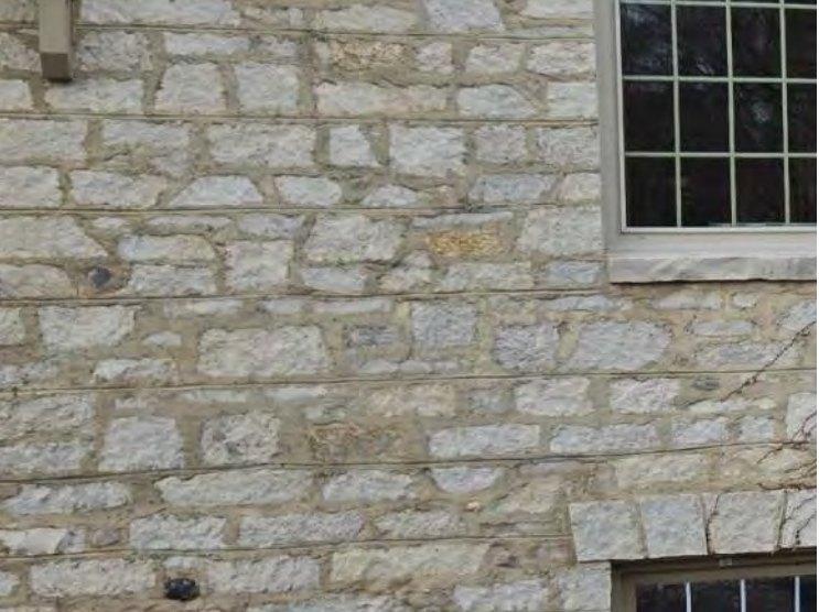
EXISTING STONE COURSING
