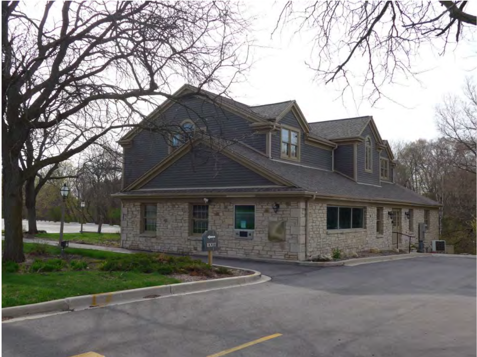
EAST BUILDING NORTH AND WEST FACADE
